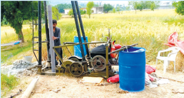
Figure 2: Step 2 (Boring)
